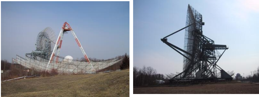
Figure 1: The 67 meter zenith antenna and the 46 meter steerable antenna. The steerable antenna is often referred to as the MISA antenna.
